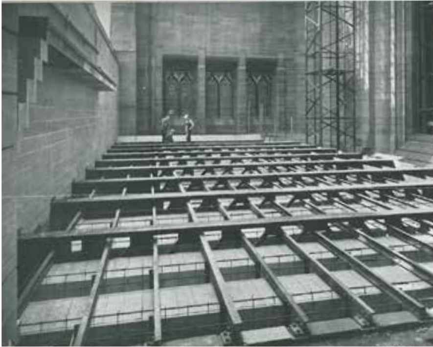
Reinforcement of the roof structure of the Welsford Porch, shown immediately before concrete is poured. [Source: Stewart Bale, reproduced in Quarterly Bulletin Vol. 4 No. 45 September 1936]
