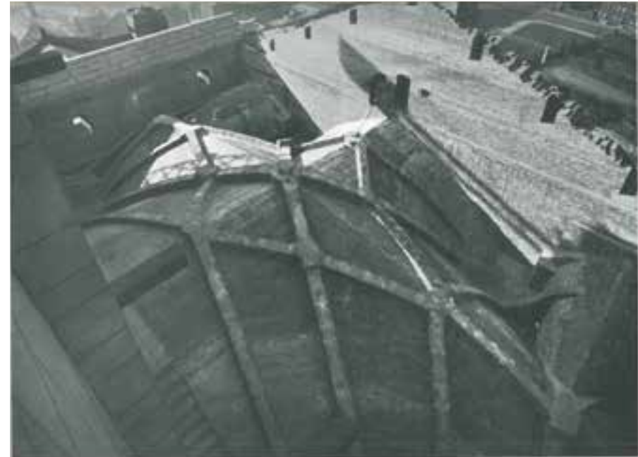
Outer leaf of the vaulting over the West Transept crossing. [Source: Stewart Bale, reproduced in Quarterly Bulletin Vol.3 No.36 June 1934]
