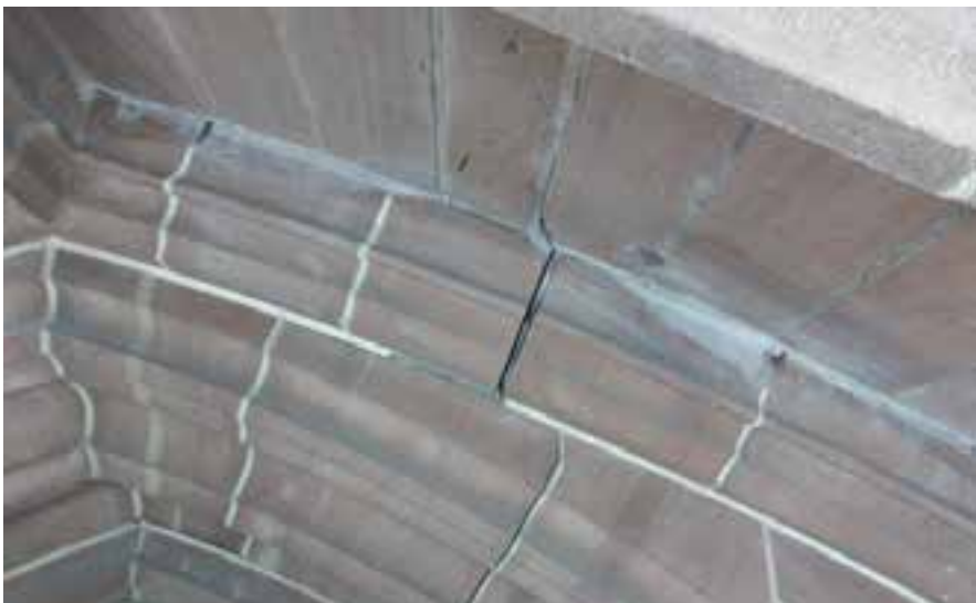
Crack in north wall of north aisle
