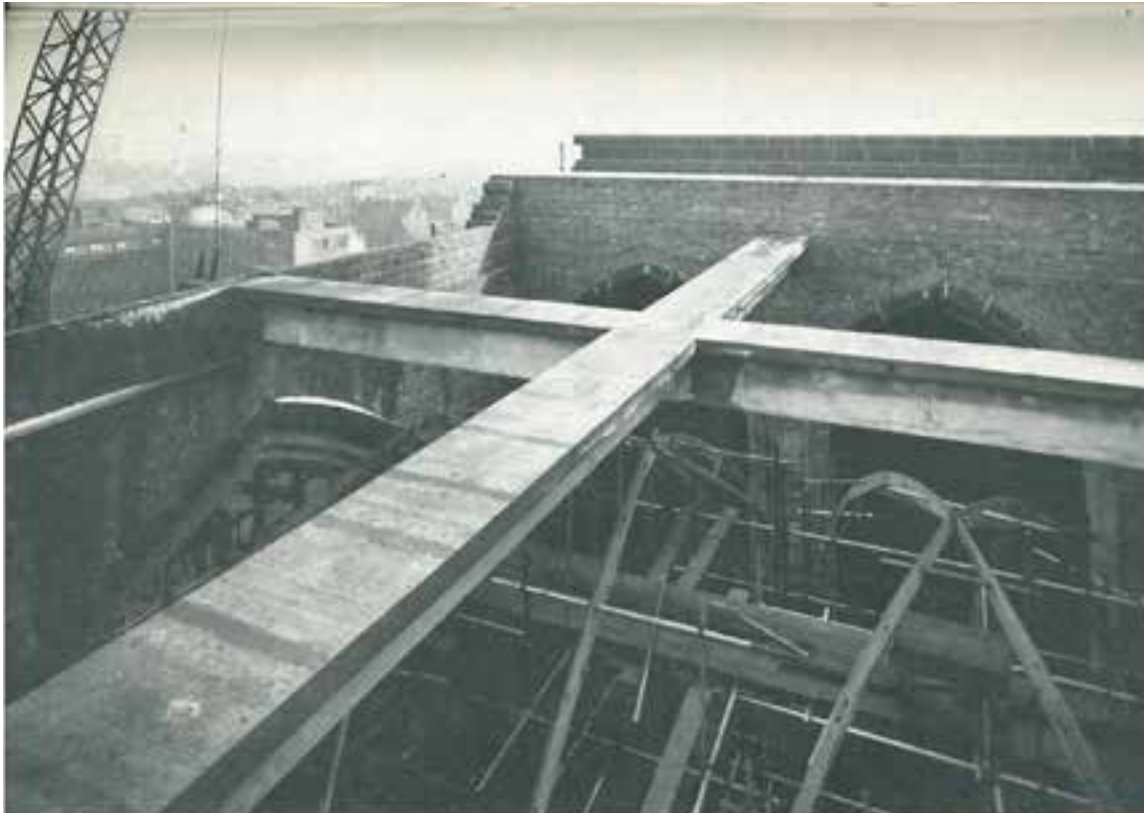
Third bay of the Nave prior to vaulting, two arches of the North Triforium are visible in the background. [Source: Elsam, Mann & Cooper Ltd., reproduced in Quarterly Bulletin Vol. 10 No.86 Dec 1964]
