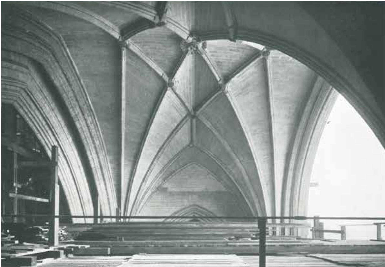
Vaulting over the West Transept crossing once the centering has been removed. [Source: Stewart Bale, reproduced in Quarterly Bulletin Vol.3 No.36 June 1934]
