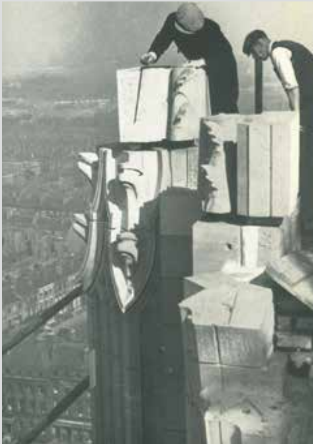
Laying stonework atop the tower [Source: Fox Films, reproduced in Quarterly Bulletin Vol.5 No.56 June 1959]
