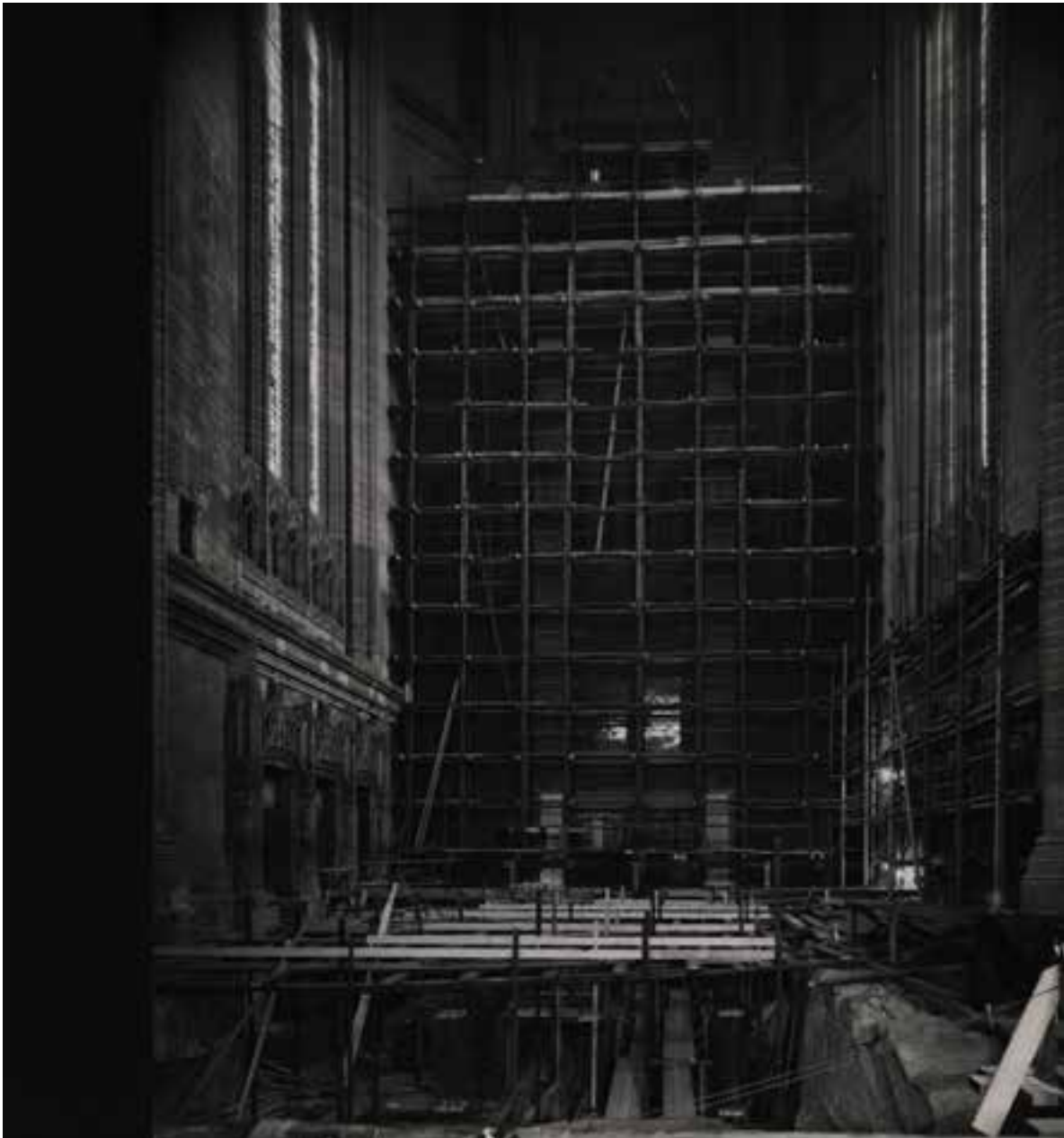
Timber scaffolding to clerestory of the Under Tower, March 1939
