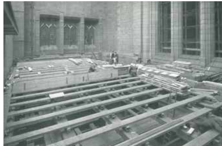
Wooden frame to take the reinforced concrete roof structure of the Welsford Porch. [Source: Stewart Bale, reproduced in Quarterly Bulletin Vol. 4 No. 44 June 1936]
