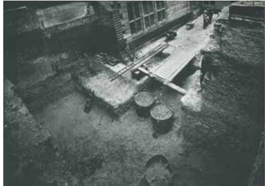
Excavation for foundations for south side of first bay of the Nave (with the basement of the unfinished Vestry visible in the background) [Source: Elsam, Mann & Cooper Ltd., reproduced in Quarterly Bulletin Vol. 7 No. 70 Dec 1948]
