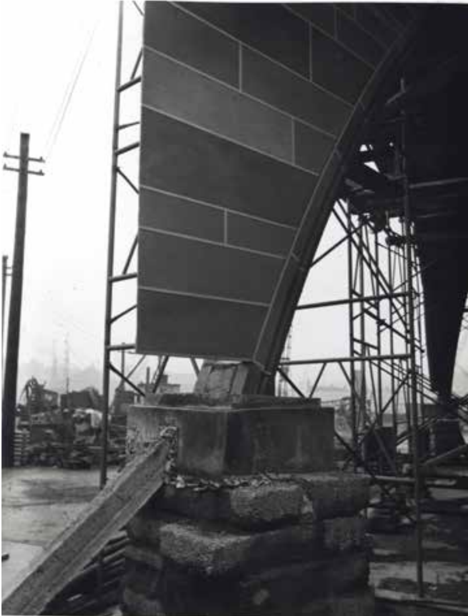
Trial setting out of arch, with painted boarding to simulate adjoining masonry (n.d.)
