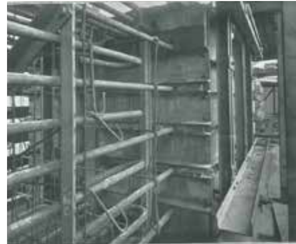
Reinforcement in the girdle [Source: Stewart Bale, reproduced in Quarterly Bulletin Vol. 4 No. 39 March 1935]
