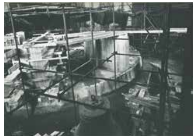
Timber shuttering for the forming the bell frame [Source: Elsam, Mann & Cooper Ltd, reproduced in Quarterly Bulletin Vol. 7 No. 72 Dec 1950]
