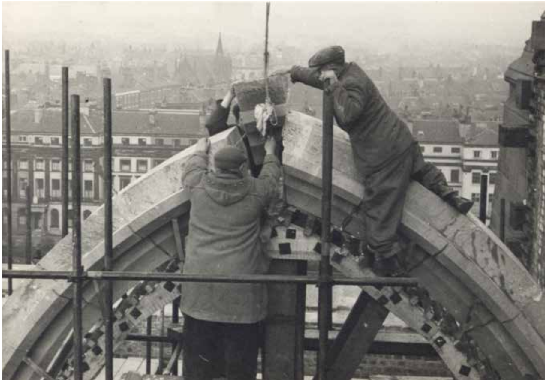
Topping out of an arch, n.d.
