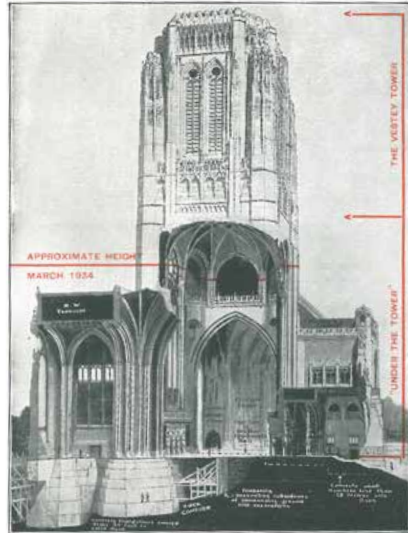
Section of the Central Space and North West Transept of the Cathedral. [Source: Quarterly Bulletin Vol. 3 No. 35 March 1934]
