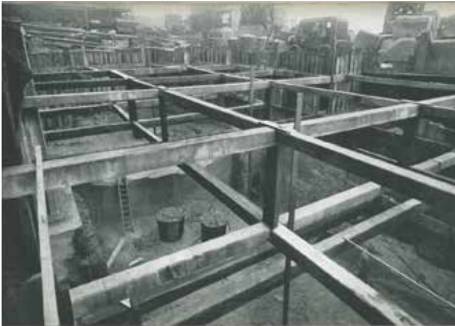
Excavation for foundations of north side of the first bay of the Nave. [Source: Elsam, Mann & Cooper Ltd., reproduced in Quarterly Bulletin Vol. 7 No. 72 Dec 1950.
