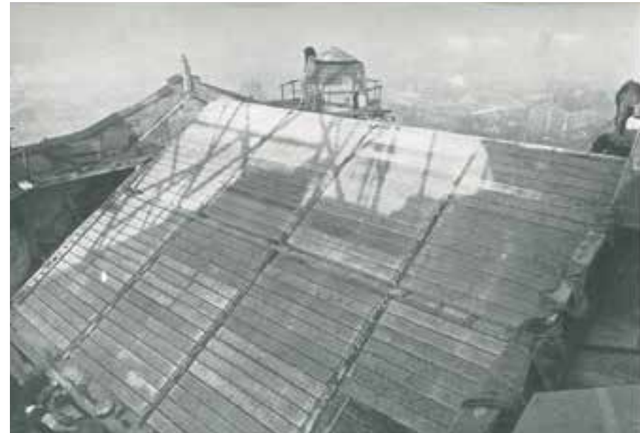
Roof structure of the south arm of the West Transept after the pre-cast concrete slabs have been slid into position, before surface will be covered with a thin layer of cement. [Source: Stewart Bale, reproduced in Quarterly Bulletin Vol. 3 No. 31 March 1933]
