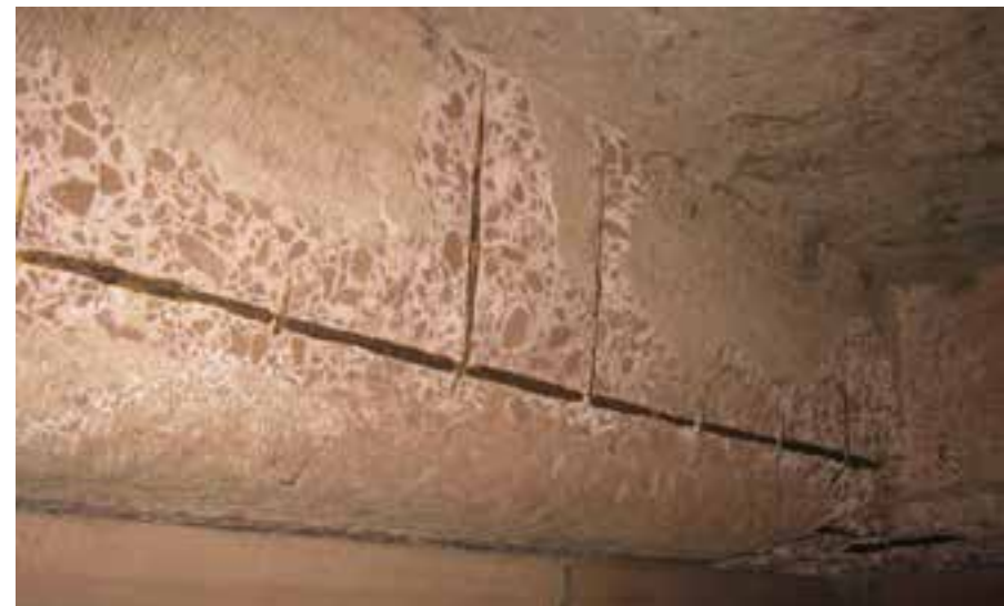
Exposed reinforcement in north west corner of Welsford Porch
