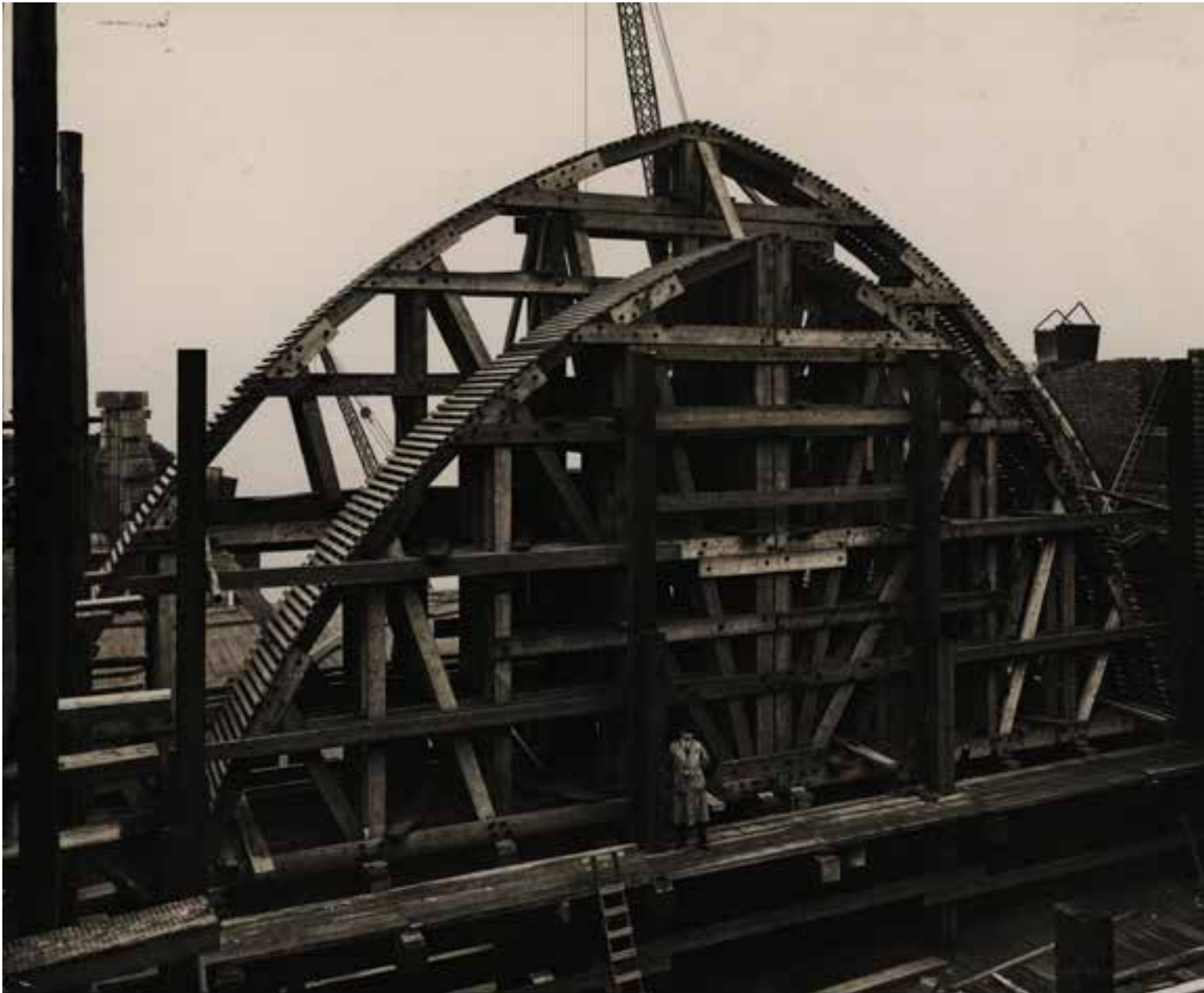
Centering for the western arch of the tower with Clerk of Works, Owen Pittaway, March 1932
