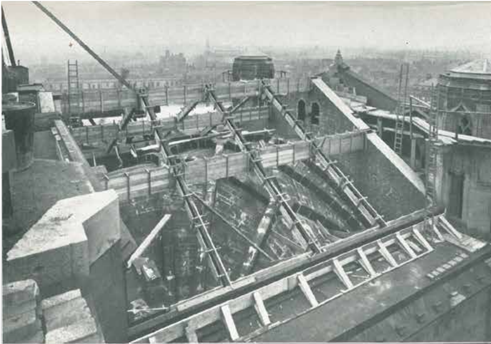
Roof structure of the north arm of the West Transept: the rolled steel is in place and ready for concrete to be poured in to form the principal rafters. [Source: Stewart Bale, reproduced in Quarterly Bulletin Vol. 3 No. 31 March 1933]
