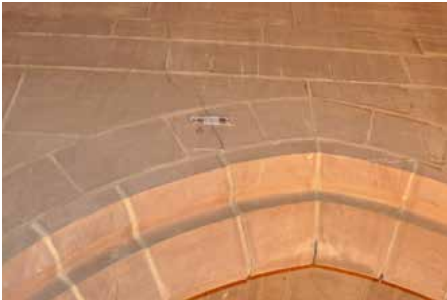
Crack in stonework in north west triforium
