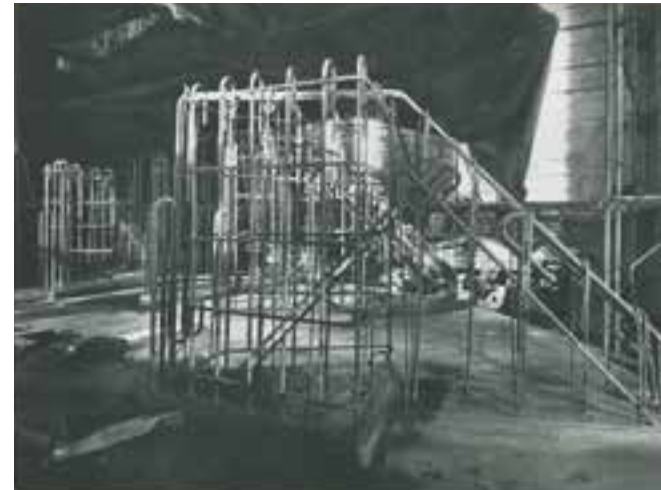
Steel reinforcements for the wedge-shaped support [Source: Elsam, Mann & Cooper Ltd, reproduced in Quarterly Bulletin Vol. 7 No. 72 Dec 1950]
